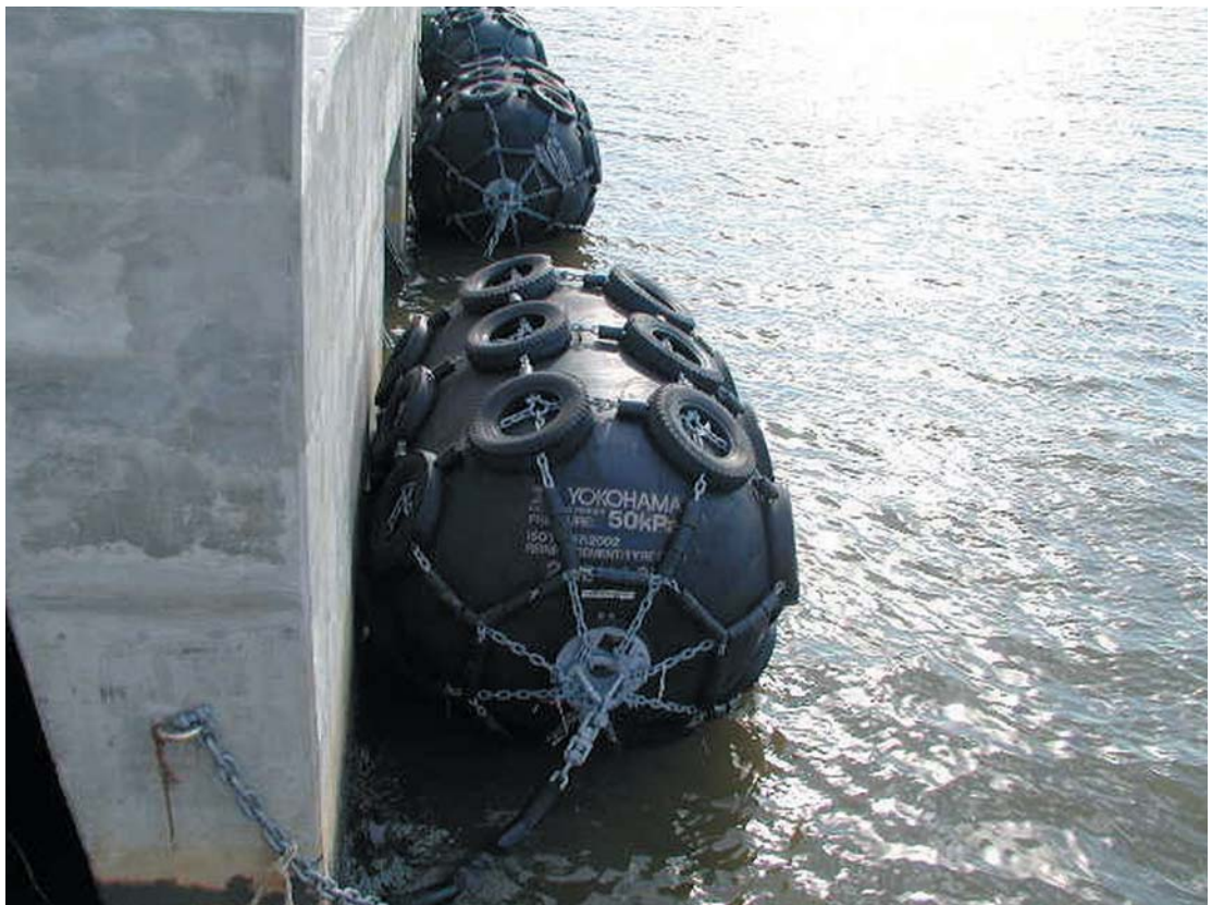
Fig.9-2 Equipments of Typical Installation for Ship-to-Jetty Applications.
