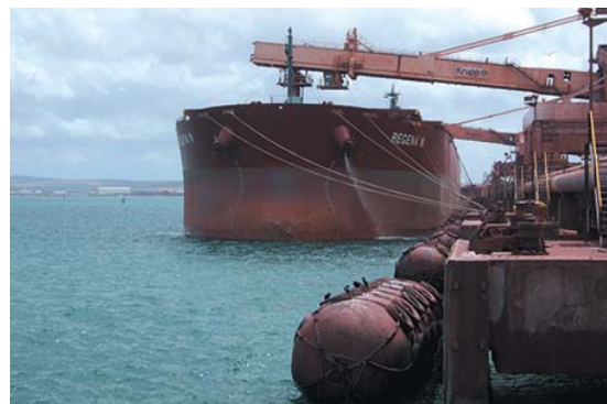
IRONSTONE TERMINAL \phi 3300 \times 10600L
