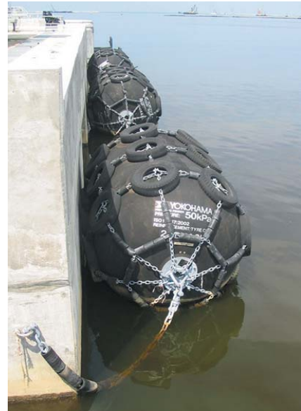
Fig.3-14 \phi 2500 \times 4000 L-P50 Yokohama Pneumatic Rubber Fenders installed at a dolphin
